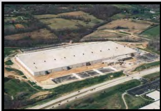
■ The recent study conducted by Oak Ridge National Laboratory shows that ballast and paver systems can save as much energy as a reflective or “cool” roof. Shown here is Toyota’s Midwest Parts Center in Hebron, KY. (Photo courtesy of Firestone Building Products Co.)
