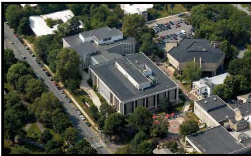
In the last 25 years, Dickinson College in Carlisle, PA, has installed more than 400,000 square feet of warranted EPDM roofing. (Photo courtesy of Carlisle SynTec Incorporated, Carlisle, PA.)
